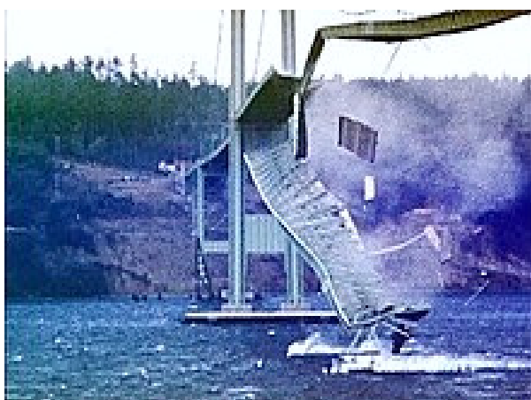
Figure 1.16(a) - Collapsing of Tacoma Narrows Bridge
